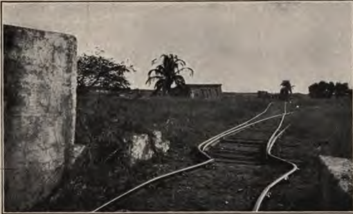
A. Subsidence of the ground with consequent tilting of buildings in the Victoria Battery, Port Royal. The kink in the railway track is over a fault.
